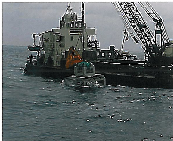
Fig. 8 Installation of Concrete Blocks
