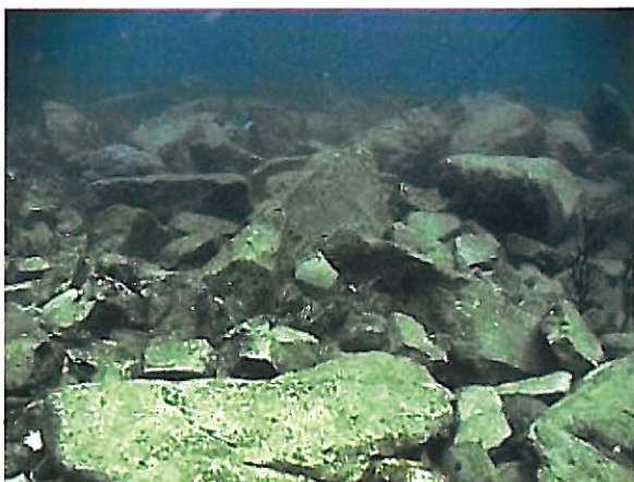
Fig. 30 Natural Stones Each natural stone weighs 500 kg - 1,000 kg and was collected from St. Vincent Island.
