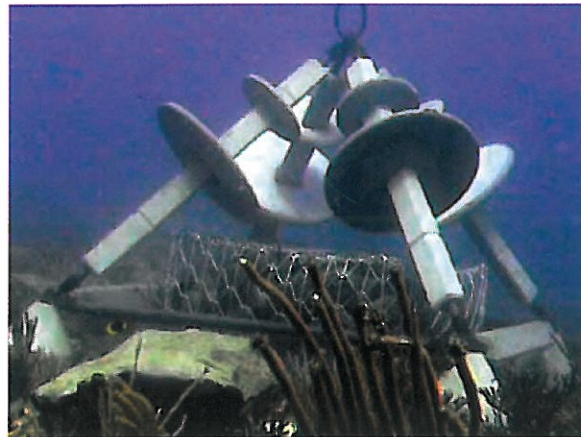
Fig. 29 Truss Reefs To make the truss reefs, parts (concrete posts, discs and gabions, etc.) manufactured in Japan were transported to St. Vincent by container ship and were assembled locally under the guidance of a Japanese engineer. The shape of complete reef is a pyramidal shape with a large surface area. The existence of large areas which are not directly exposed to the water current as well as hiding areas creates a habitat for organisms which are eaten by fish. As such, this type of reef promises a high fish gathering effect and shelter effect for long residence by fish and the favourable growth of young fish. For the purpose of attracting lobsters, the bottoms of these truss reefs were combined with a gabion basket which was filled with small natural stones.
