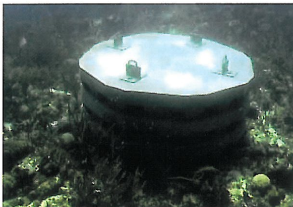
Fig. 31 Lobster Reefs A lobster reef has layers of concrete discs with a slit for lobsters to hide between the discs. All of the discs except the top disc have a centre hole to allow the lobsters to move from one floor to another. The slit size corresponds to the size of adult lobsters which inhabit that area.
