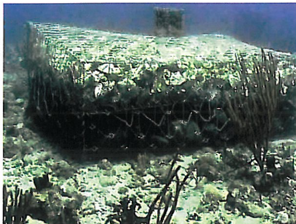
Fig. 28 Newkarus Units Newkarus units are cube-type mesh baskets made of steel wires coated with vaporised aluminium. For the experiment, these units were filled with small natural stones and local dumped conch shells. The small gaps created by the small natural stones and conch shells can be used as shelters for young lobsters and small fish. The utilization of conch shells was decided partly because of the expectation for the attachment of organisms which can be eaten by fish and partly in an attempt to recycle waste materials.
